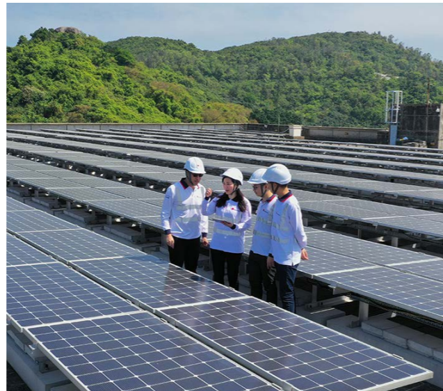
200 kW capacity solar installation at Gammon Technology Park in Tseung Kwan O.
