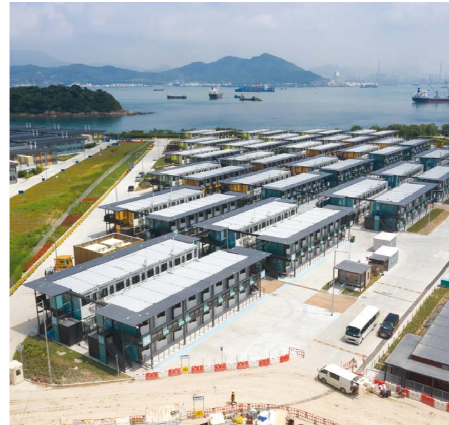
Penny's Bay quarantine facilities, where we monitored all phases of the MiC works using digital solutions that fed real-time data to the Hong Kong construction industry's first 5G Smart Control Centre.
