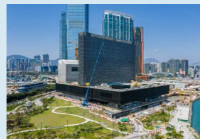
High levels of precision achieved quality finishes as well as a reduced potential for waste on our M+ Museum project.
